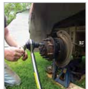
Torque multiplier used for lug nuts
